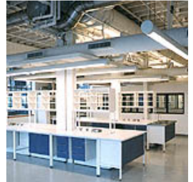
The lab spaces of the Triangle Biotechnology Center are furnished with modular, Scandinavian-designed casework. Photo: Michael Traister
